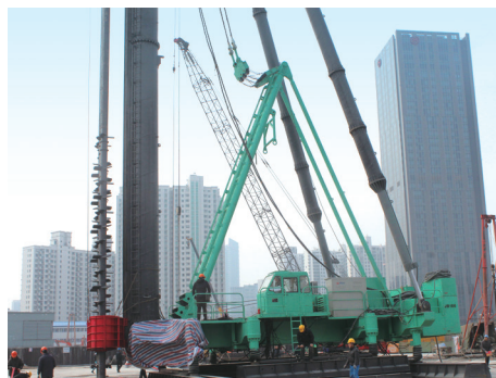
上海海伦路工地 Hailun Road, Shanghai
