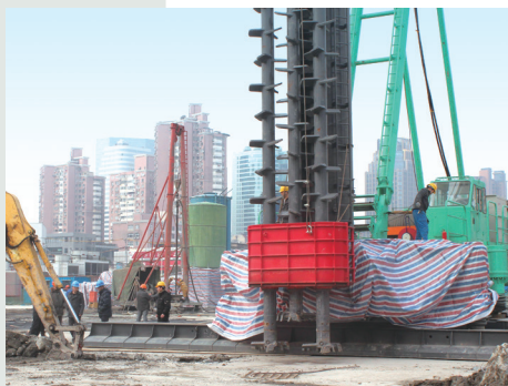
上海海伦路工地 Hailun Road, Shanghai
