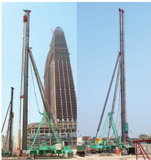
苏州东方之门工地 The Gate of the Orient, Suzhou
