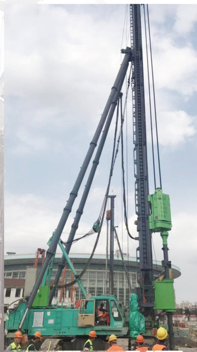
挂静钻根植工法钻机施工 Pre-bored Pre-cast Piling attached to SPR135
