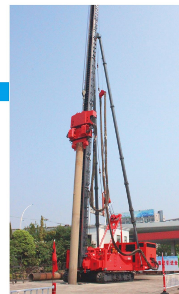
挂液压振动锤施工 Hydraulic Vibratory Hammer attached to SPR115
