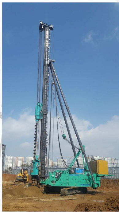
挂双动力头钻机施工 Dual Power Drilling Rig attached to SPR115
