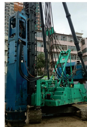
挂液压锤施工 Hydraulic Hammer attached to SPR115
