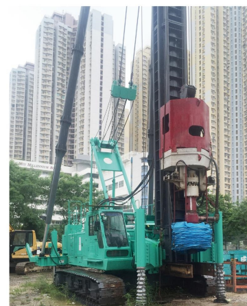
挂入岩钻机施工 Auger attached to SPR115
