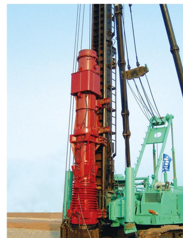
挂筒式柴油锤施工 Diesel Pile Hammer attached to SPR115
